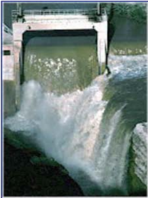
Hydroelectric dam on the Virgin River.
